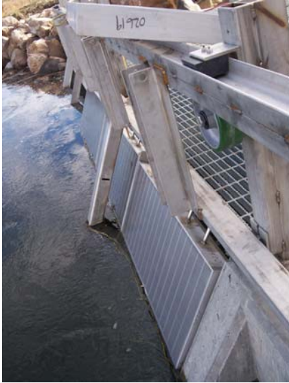
Motor drive fish screen designed to protect fish from irrigation pumps.
