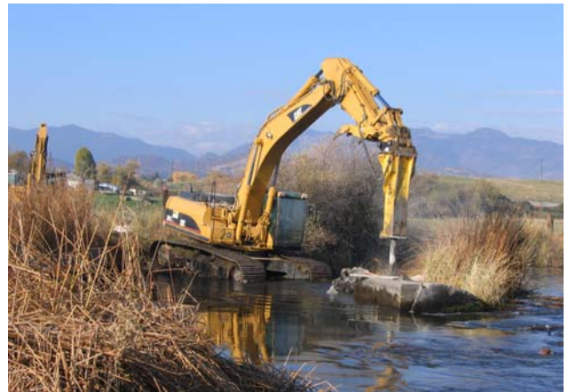
Removal of the Araujo Dam (Oct 2007)
