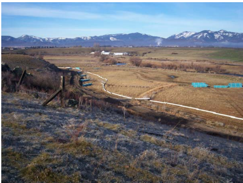
Installation of pipeline to replace earthen ditches.
