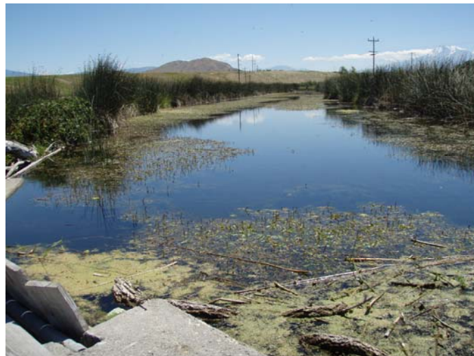
Ponded water upstream of the dam creates poor water quality in the river.
