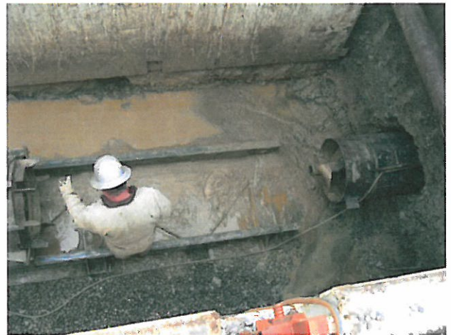
Boring underneath a Siskiyou County Road, railroad track and fiberoptic line for the Upper South Ditch pipeline.
