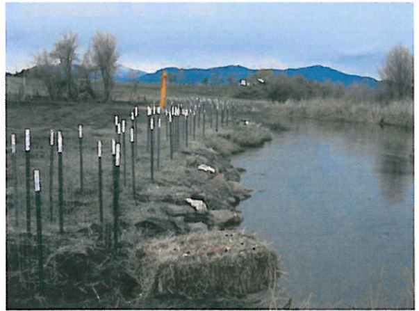
Revegetation of disturbed streambanks both upstream and downstream of the SRWA fish screen. The t-posts support wire cages placed around willow plantings to prevent damage from local beavers.
