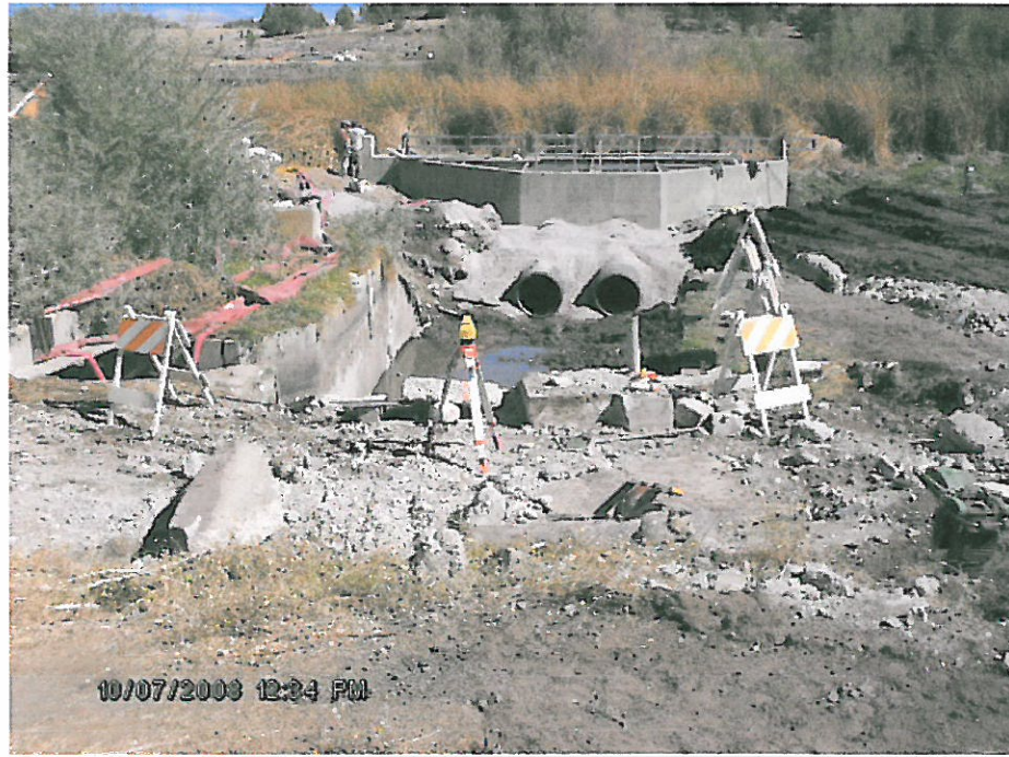
Backfill of fish screen and demolished pump station.
