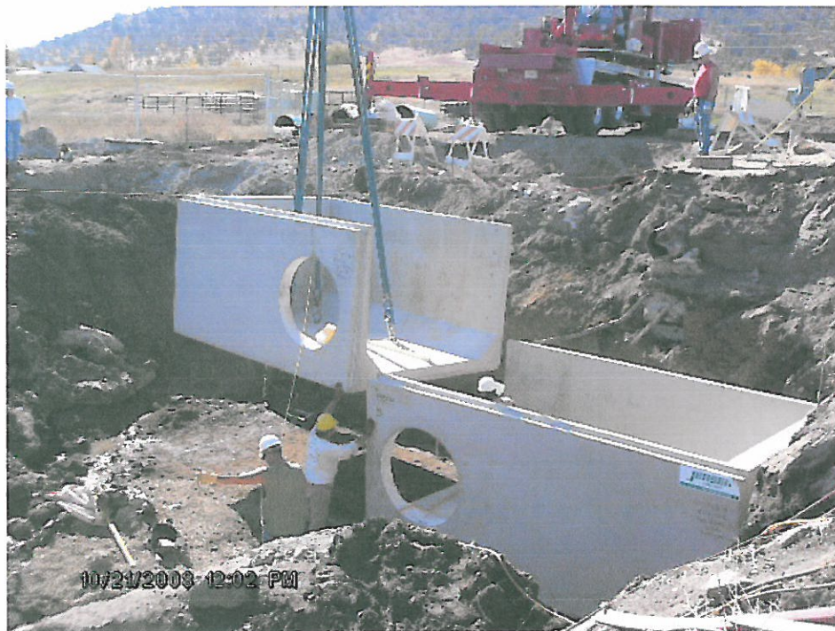
Installation of wetwells.
