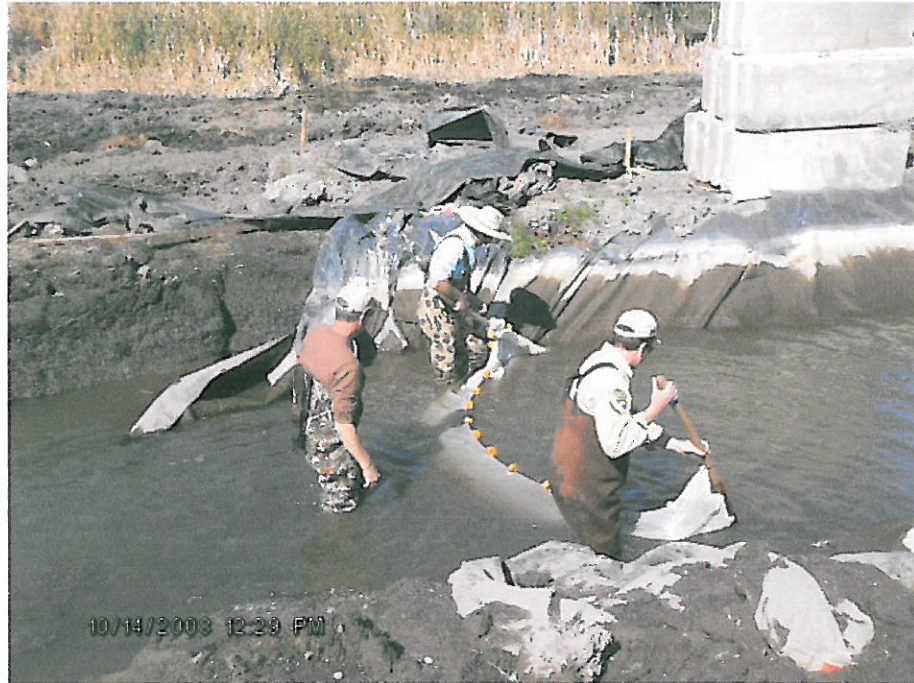
Fish salvage by CDFG in the temporary bypass channel before backfilling.
