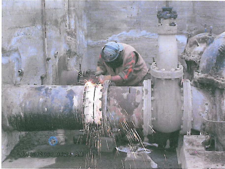
Demolition of the pump station and dismantling of the old pumps.
