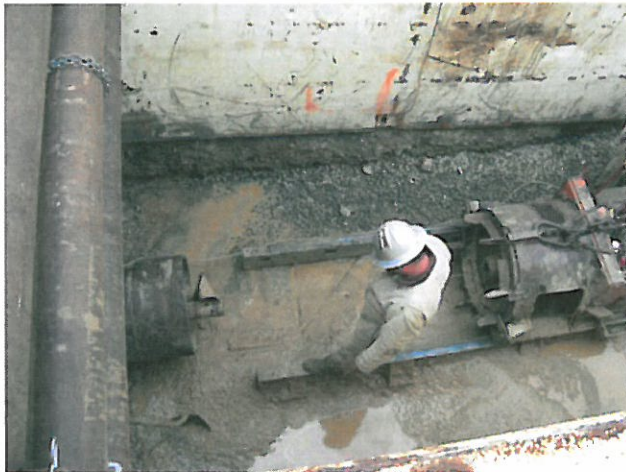
Boring underneath a Siskiyou County Road, railroad track and fiberoptic line for the Upper South Ditch pipeline.
