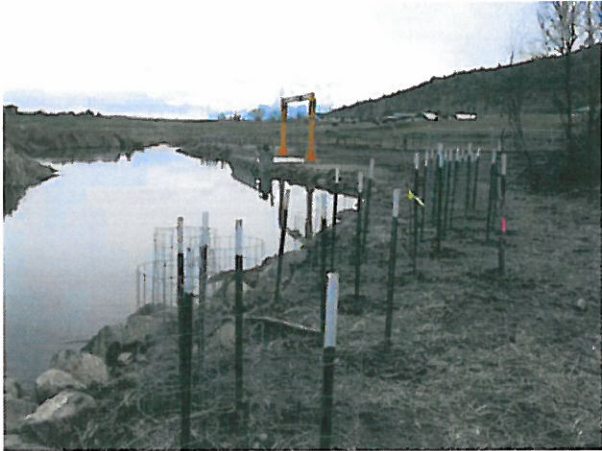
Revegetation of disturbed streambanks both upstream and downstream of the SRWA fish screen. The t-posts support wire cages placed around willow plantings to prevent damage from local beavers.
