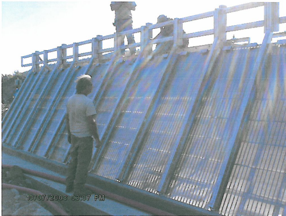
Completion of the fish screen's brush arm assembly.
